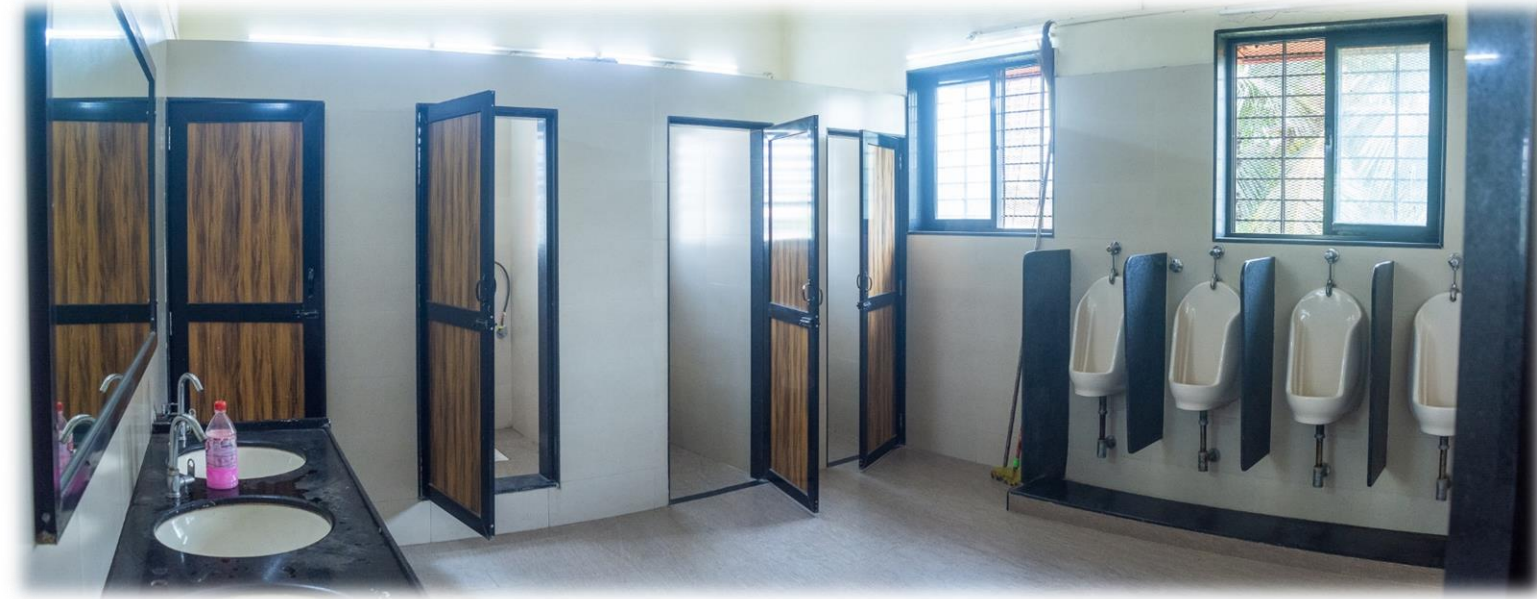
Boys Toilet – Fourth Floor
