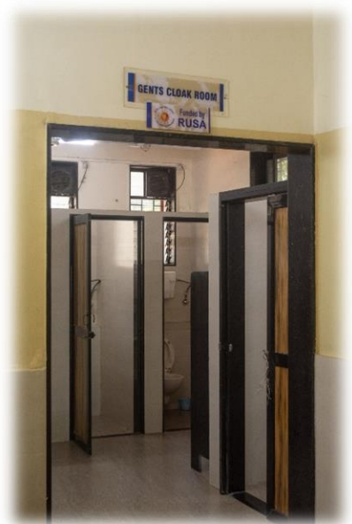
Boys Toilet – First Floor
